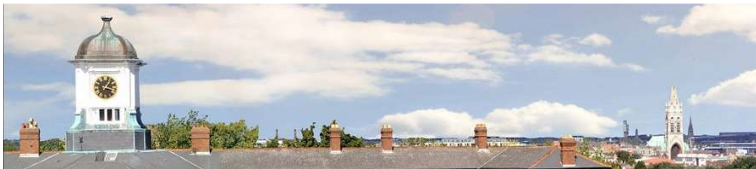
Pictured above: South Circular Road Campus
