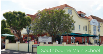
Southbourne Main School
