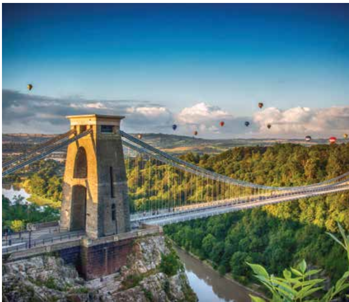
Clifton Suspension Bridge, Bristol
