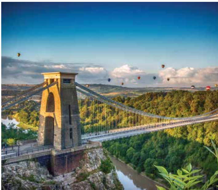
Clifton Suspension Bridge, Bristol
