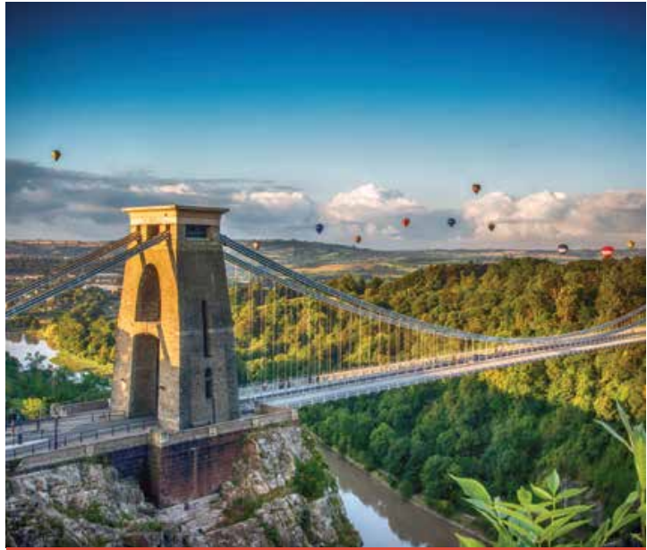
Clifton Suspension Bridge, Bristol
