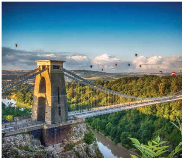
Clifton Suspension Bridge, Bristol
