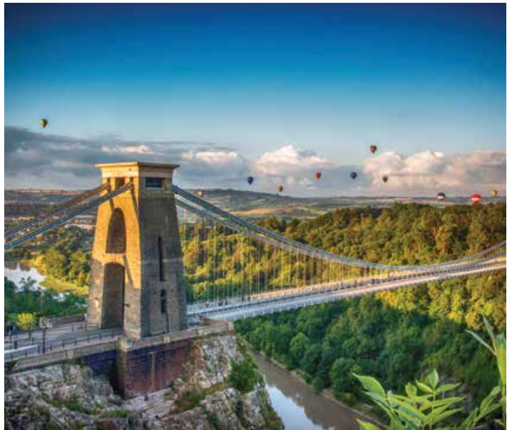
Clifton Suspension Bridge, Bristol
