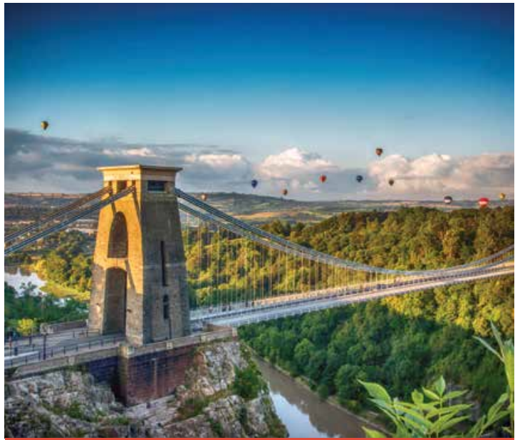
Clifton Suspension Bridge, Bristol
