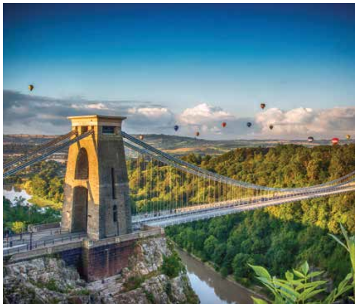
Clifton Suspension Bridge, Bristol
