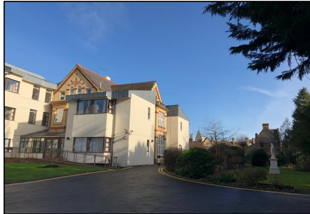
The exterior of Mary Ward House residential accommodation
