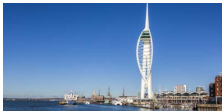
Spinnaker Tower - Portsmouth
